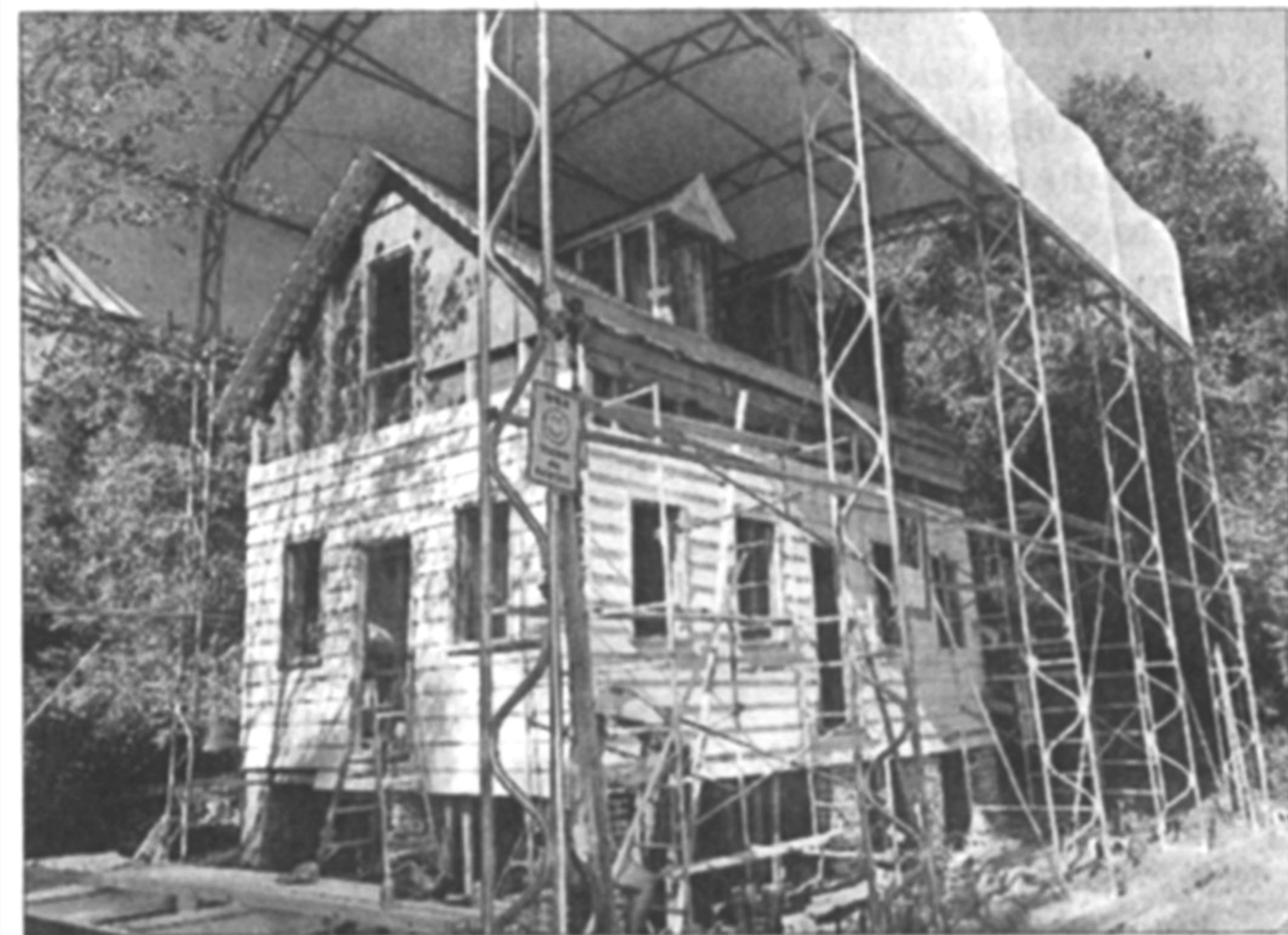
The Edisto Island Open Land Trust erected this tent structure in 2017 to protect the Henry Hutchinson House while it awaited stabilization. That work is largely done, and it plans to sell the tent.
